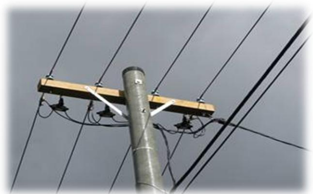
Auditing O/H construction fibreglass pole
