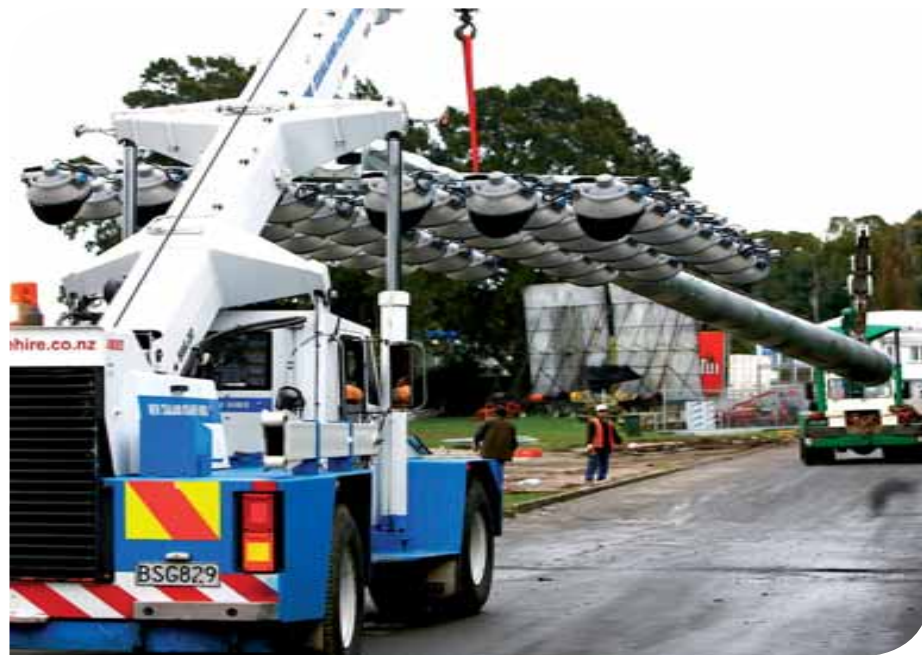
Moving one of the four temporary towers into place
